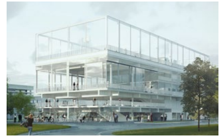
“Public Condenser – Low-cost flexible university building” by Muoto architectes, Paris, France (Silver Award 2014 Europe).
